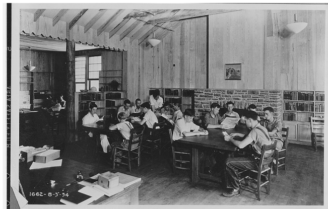
Miscellaneous design. Libraries in rural areas are among the great needs of the Tennessee Valley. The one shown in this photograph was built and equipped with the assistance of work relief labor out of primitive local materials. [between 1933 and 1945]
