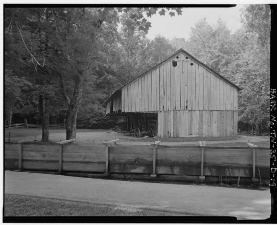
19. Cantilevered barn in Cades Cove looking SSW. HAER TENN,78-GAT.V,6D-19 from Great Smoky Mountains National Park Roads & Bridges, Cades Cove Road & Laurel Creek Road, From Townsend Wye to Cades Cove, Gatlinburg vicinity, Sevier County, TN. [after 1968]
