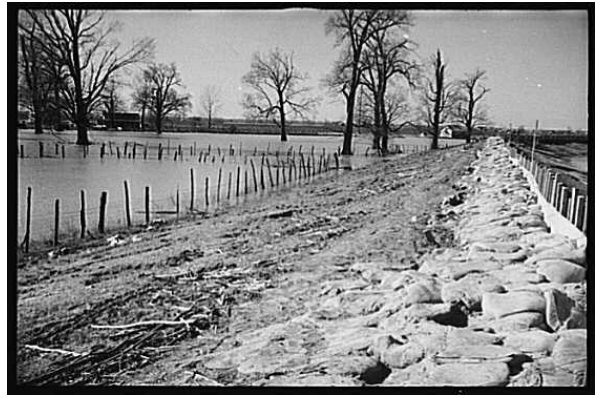
The Bessie Levee augmented with sand bags during the 1937 flood. Near Tiptonville, Tennessee.
