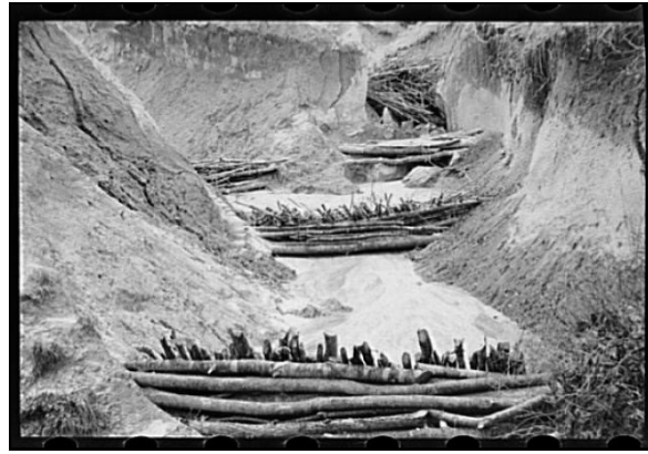
Erosion control on Natchez Trace Project near Lexington, Tennessee. [1936]
