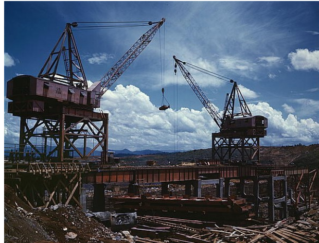
Construction work at the TVA's Douglas Dam, Tenn. [1942]
